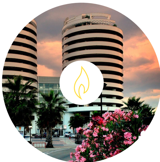
GAS PIPING SYSTEM in luxury residence of Torri Camuzzi, Pescara, Italy
