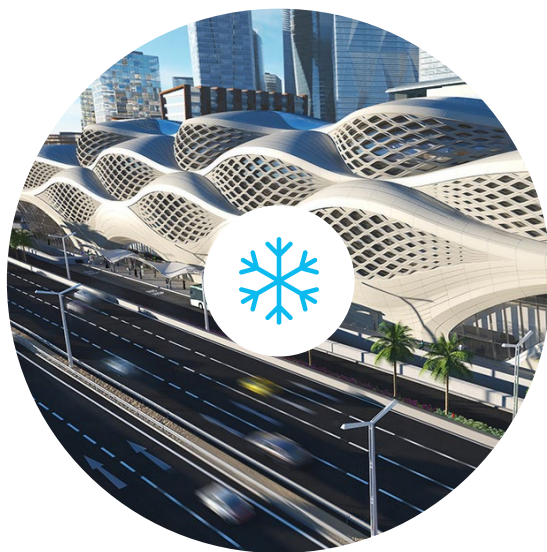
King Abdullah metro station, Riyadh, Saudi Arabia UNDERFLOOR COOLING systems
