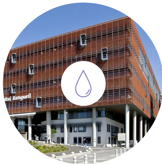
SANITARY PE-Xb pipes, Hospital of Toulouse, France
