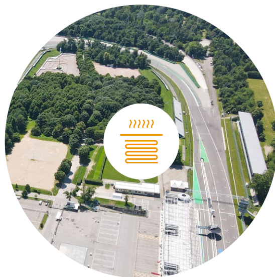
PE-Xb HEATING pipes under the racing circuit in Monza, Italy
